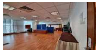
Renovation of Office Space and Other Related Works at the Examination and Certification Unit, Training Management Division, MOH
